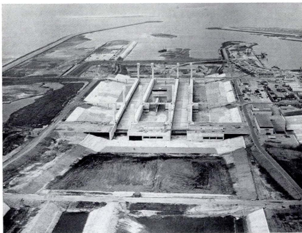
Photo 13. General view of the Kreekrak lock system just before the flooding of the construction site. The concrete work has been completed. The forebays are being dredged to the requisite depth.
