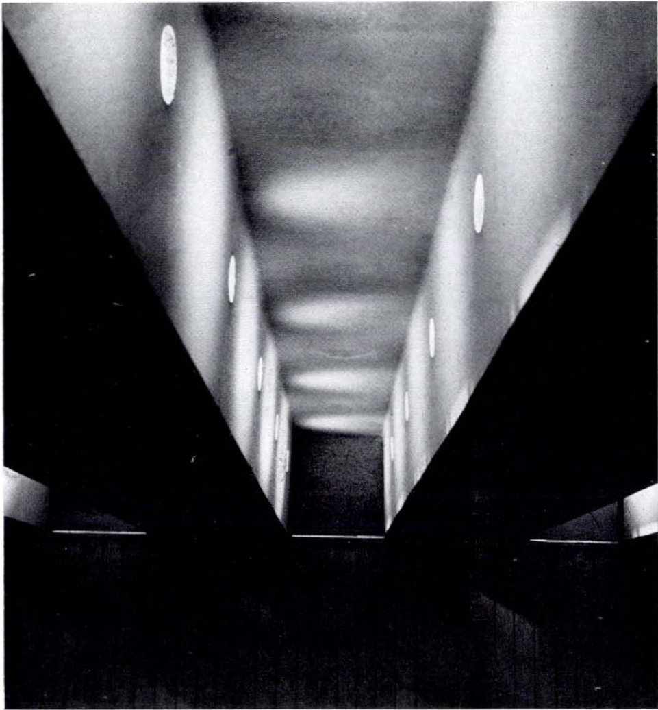
Photo 3. Detail of floor beam.
