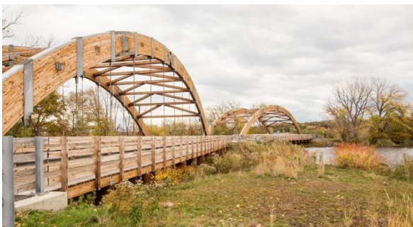
Overpeck Park Entrance Bridges, 63 Teaneck, New Jersey, 2012.
