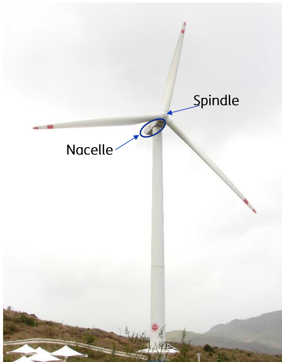
Figure 1.1 Wind turbine generator 11 and location of the nacelle and spindle. The nacelle is regarded as the main source of EMI.
