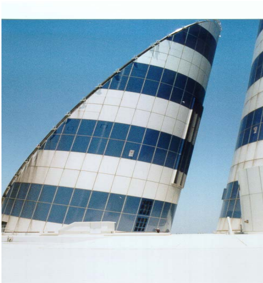
Stack at Tokyo Bay Tunnel, Japan
