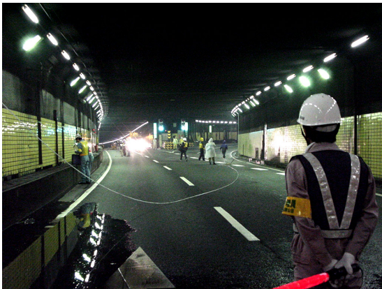
Figure D-45 Preparation for sprinkler test in branch section
