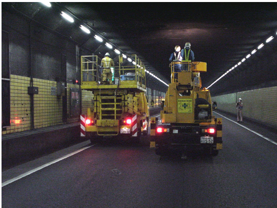
Figure D-13 Inspection of light armatures and ceiling
