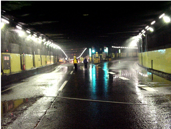
Figure D-51 End sprinkler test for branch section
