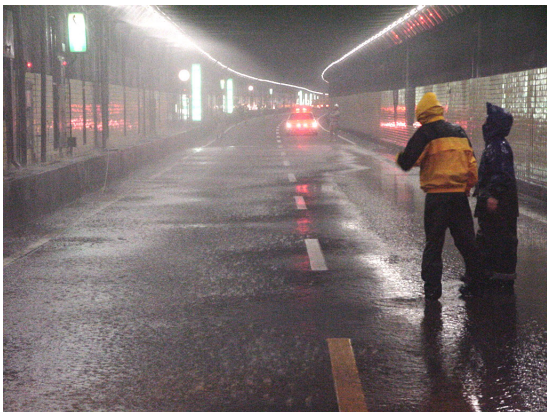
Figure D-33 Turning down sprinklers
