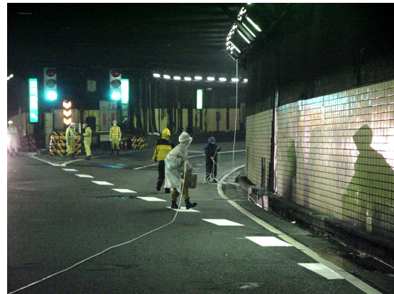
Figure D-46 Preparation of water pressure measurement
