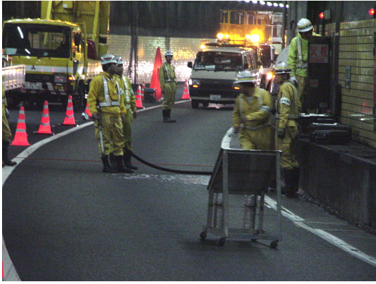
Figure D-9 Preparation for fire hose inspection
