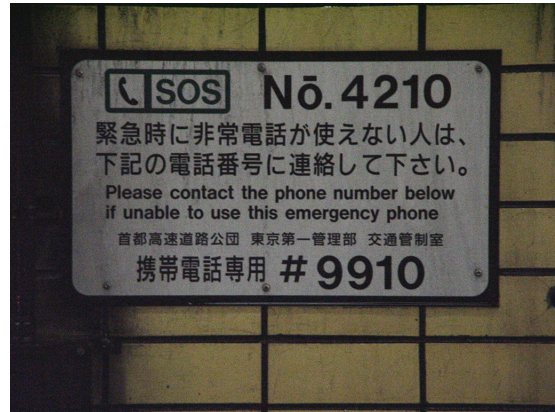
Figure D-44 Message board for emergency telephone
