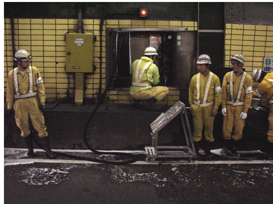
Figure D-12 Cleaning of SOS station
