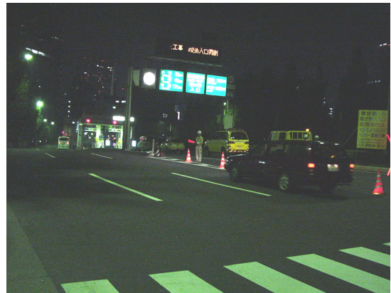
Figure D-4 Message boards in front of tunnel entrance (toll booths): "Entrance closed due to works"
