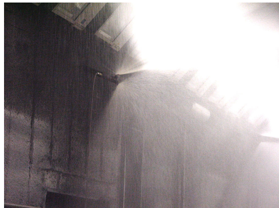
Figure D-28 Detail of sprinkler head
