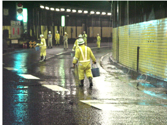
Figure D-52 Clean up after sprinkler test
