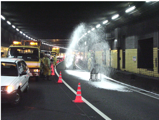
Figure D-11 Fire hose spray inspection
