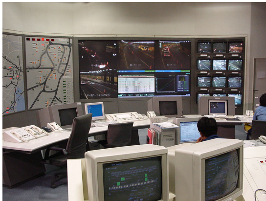
Figure D-5 Miyakezaka Facility Operation Office
