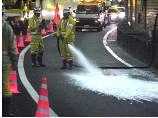
Figure D-10 Fire hose inspection
