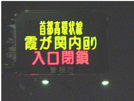
Figure D-3 Message board at road towards tunnel: "Inner Circular Route closed to traffic"
